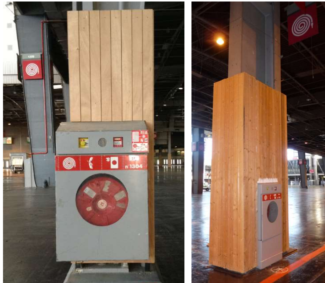
FIRE HOSE REEL
